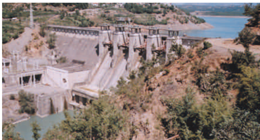
Concrete dam at the Ulza hydropower plant.
