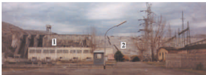
Vau Dejes hydroelectric power plant dam. (1) Concrete section; (2) gravel-fill section.
